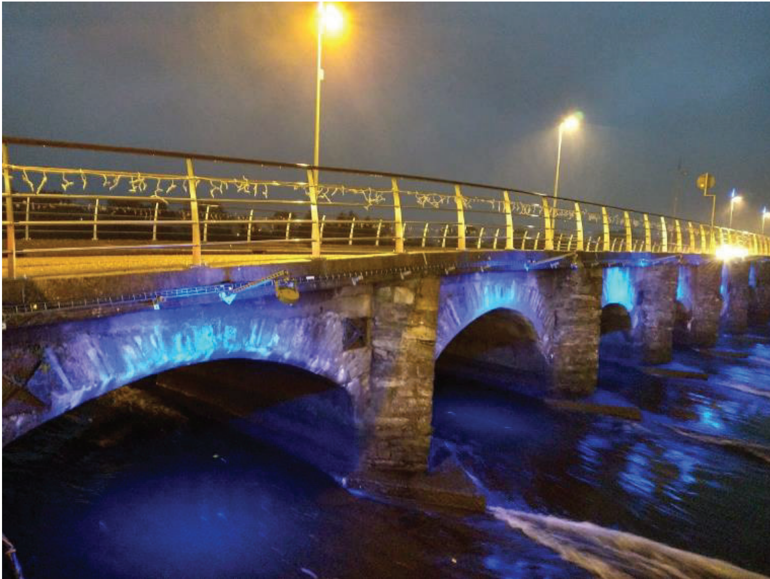
Existing lighting of the bridge. Most illumination is to the east while bats roost to the west. Nonetheless, lighting has increased considerably since 2017
