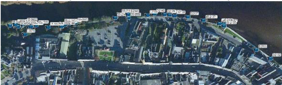
Close-up along the Avoca River to the west of Arklow Bridge
