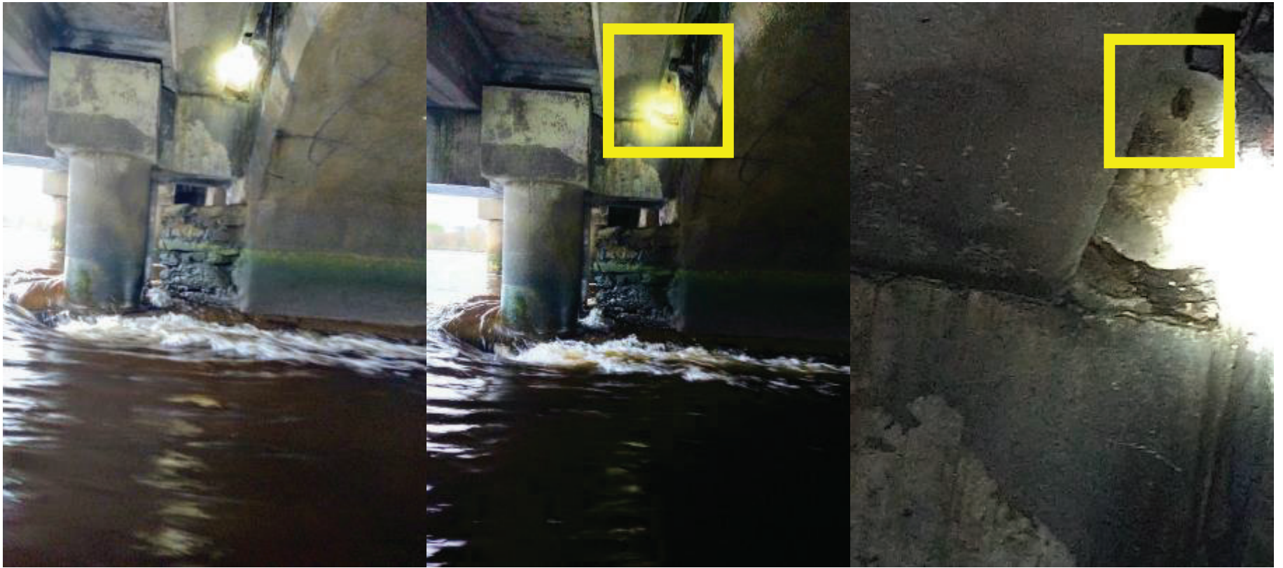
Daubenton's bat on the southernmost arch of Arklow Bridge November 17 th , 2020
